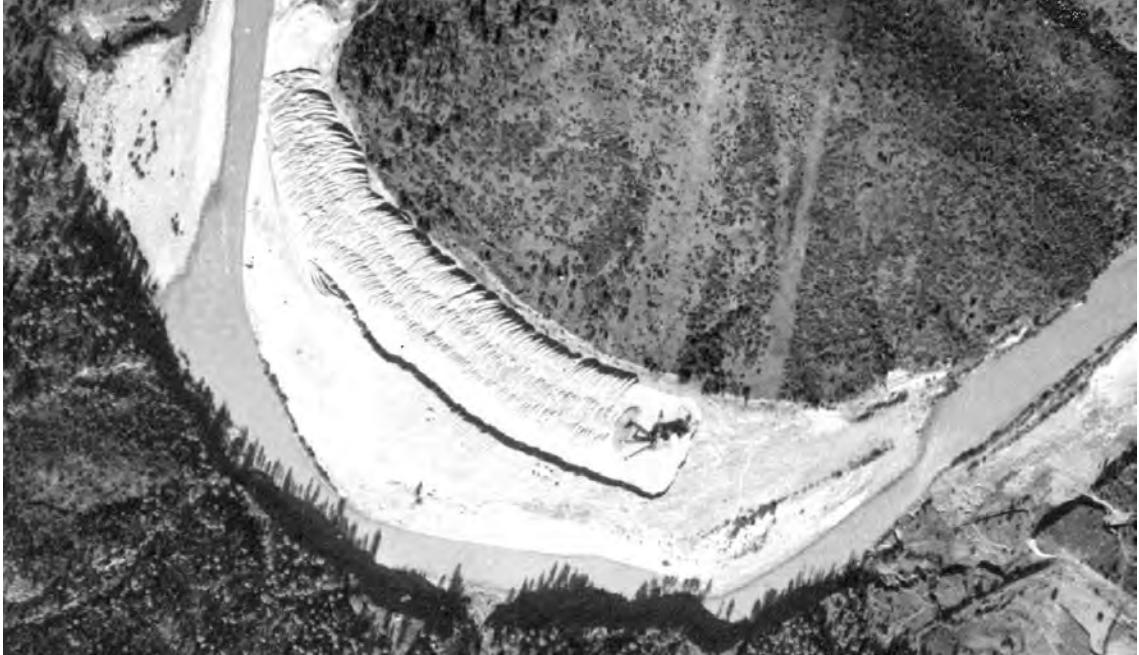
Figure 1.3. Dredger forming high tailings berm out of a mining-waste point bar at Rose Bar on 10/21/1937. (Photo from the California Transportation State Archive).
