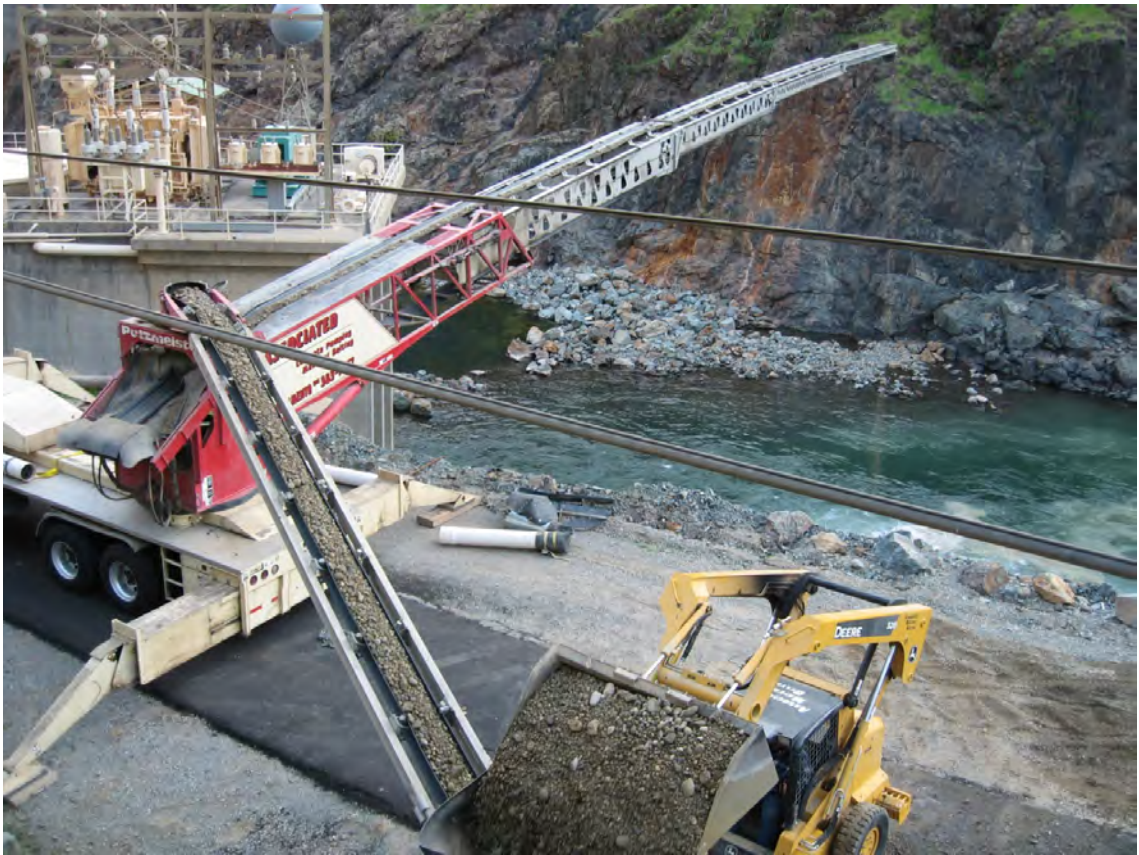
Figure 2.3. Gravel injection on November 29, 2007. Gravel pile is located in zone of aeration downstream of the Narrows II powerhouse.
