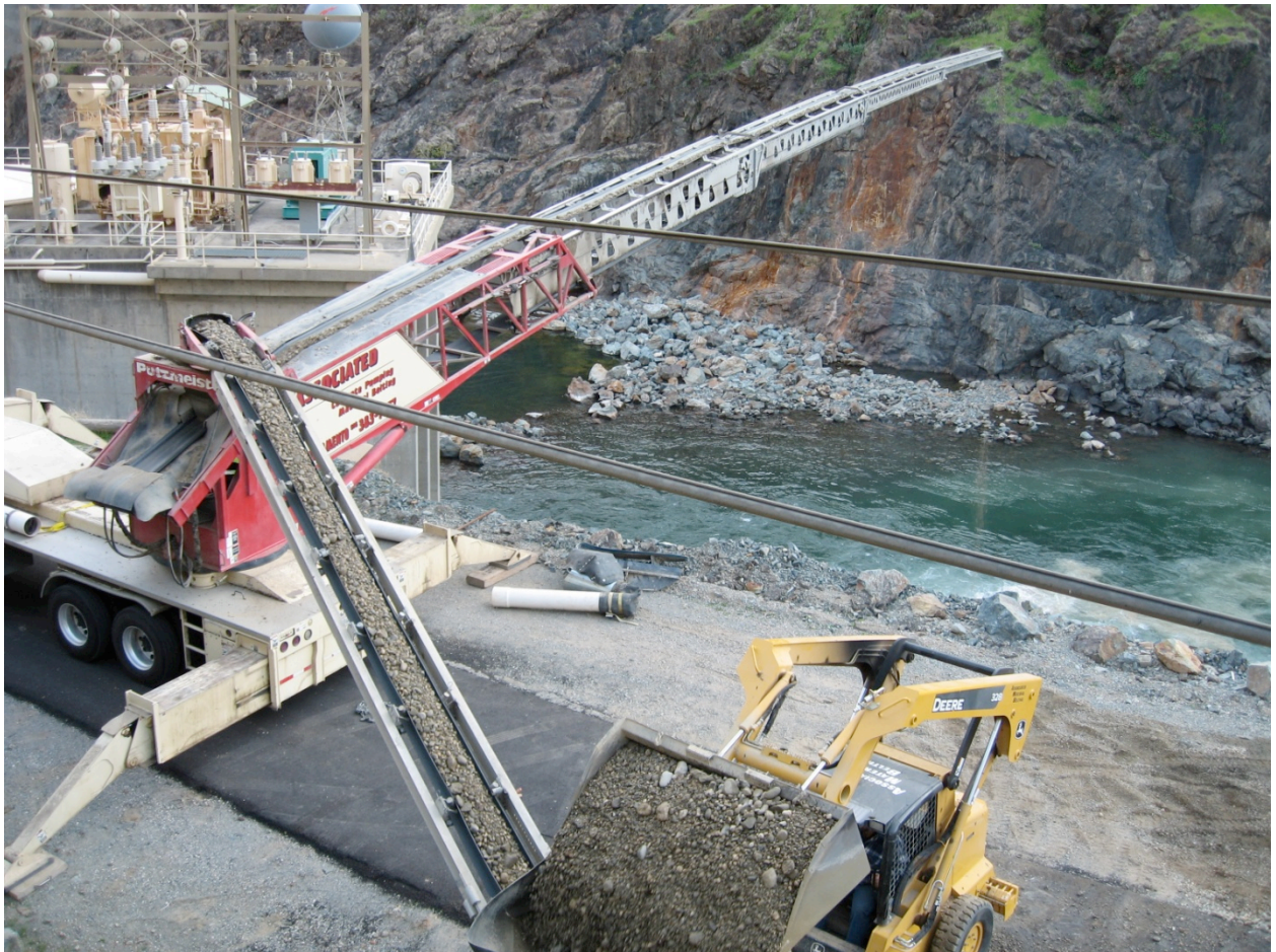
Figure 6. Gravel injection on November 29, 2007. Gravel pile is located in zone of aeration downstream of the Narrows II powerhouse.
