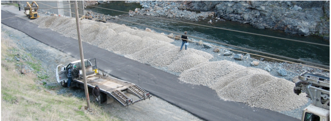
Figure 5. 500 short tons of triple-washed gravel prior to injection.
