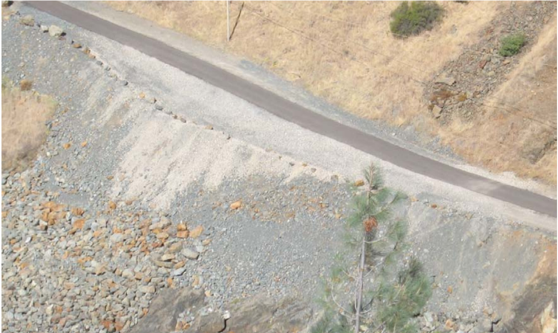
Figure 2.4. Photo of stockpiled gravel/cobble left on the parking area and hillside after the 2007 pilot injection.
