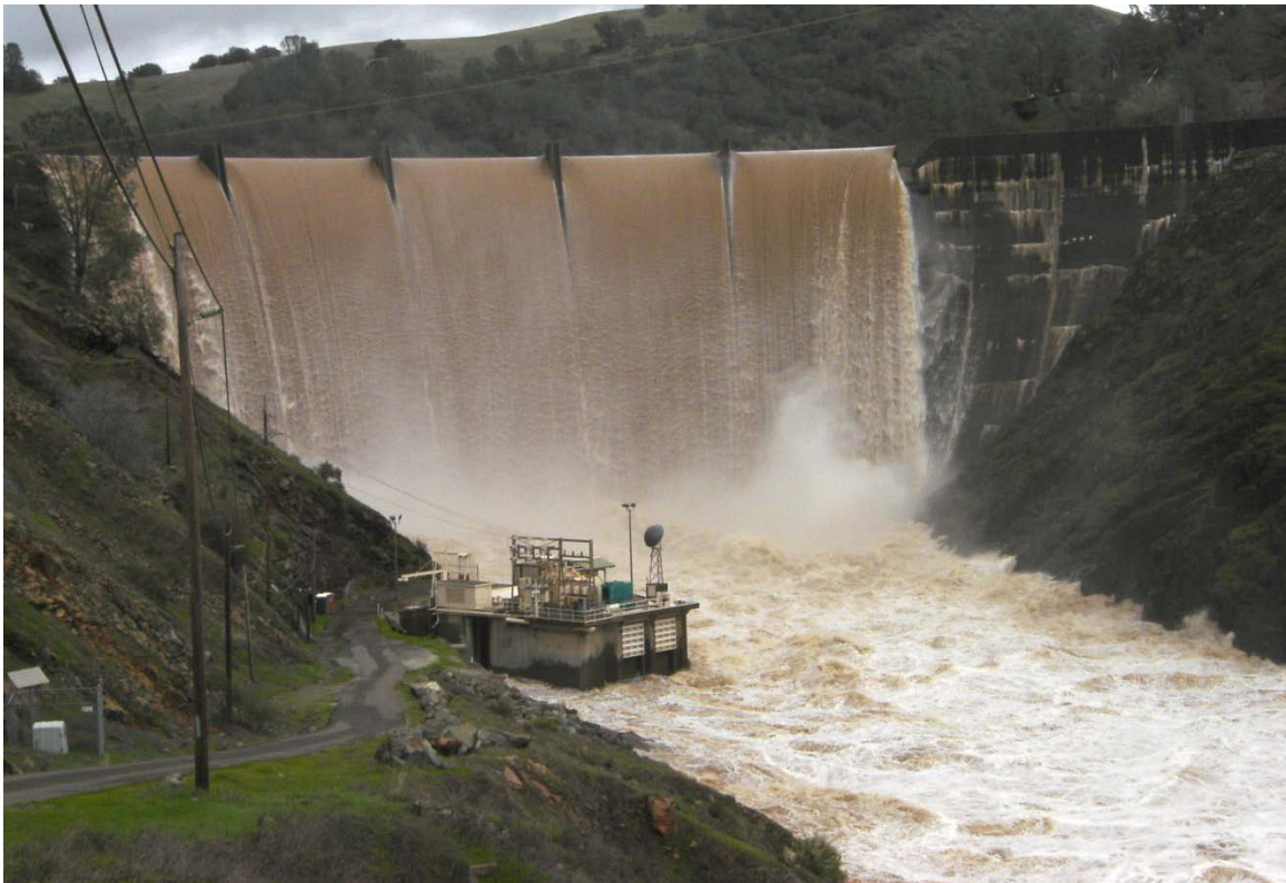
Figure 4.1. Photo of the New Year's 2006 flood drowning the area where a road would have to be built to use trucks and front loaders as the delivery method for gravel/cobble augmentation. Aggressive velocities were evident all along the north bank.
