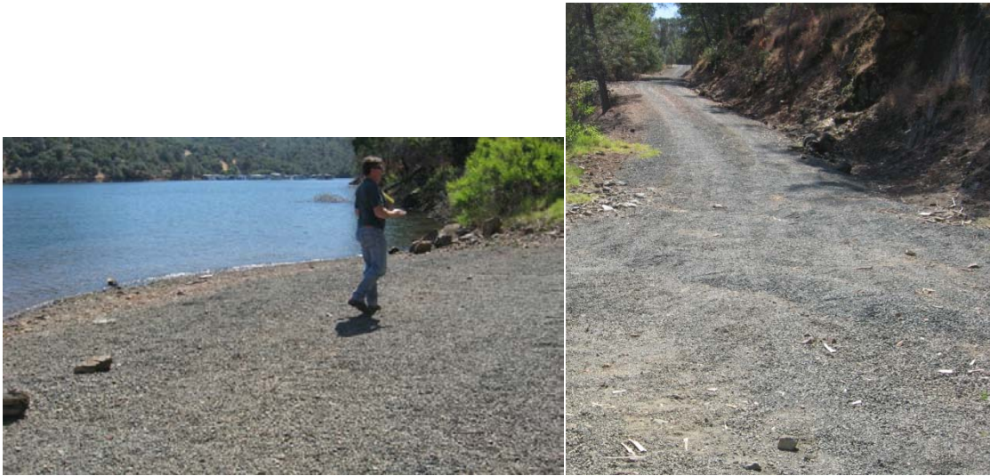
Figure 4.3. Landing area at the water's edge of Englebright reservoir (left) and gravel road leading up to the hillcrest (right).
