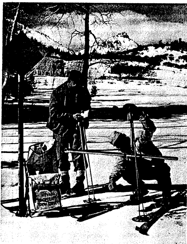
FIGURE 1.22.—Measuring water equivalent of snow by weighing the core taken by the sampler.
