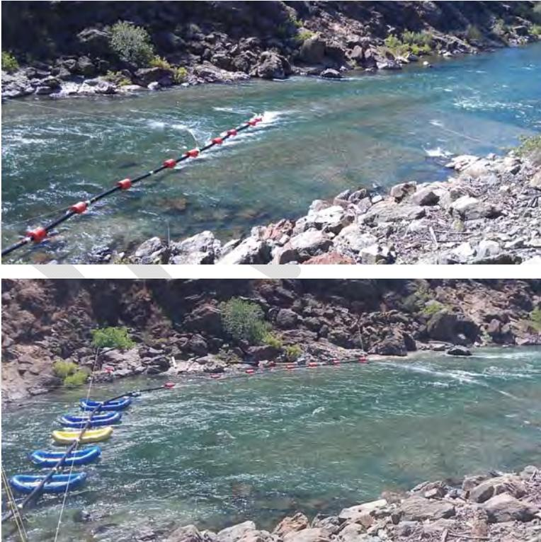
**Figure 3. The sluice pipe outlet in the river without barges and only a limited cableway (top) showing that the pipe is pushed downstream by the flow and there is less control on cobble/gravel placement. When barges and cableway are used (bottom) there is excellent control on pipe length and positioning.**
