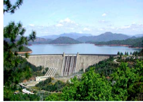
Present Shasta Dam
